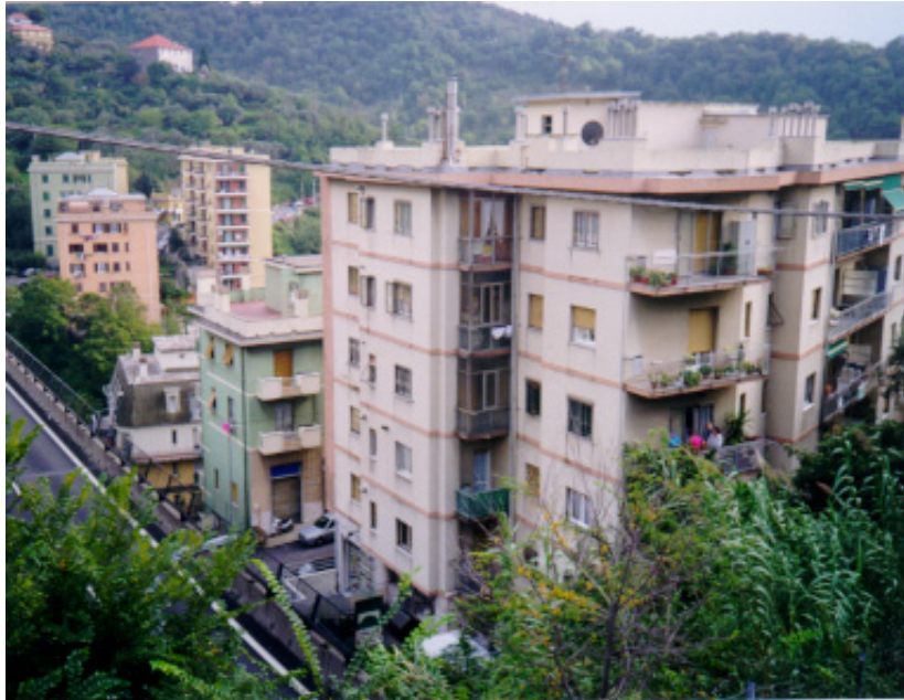
Figure 3: High Sound Insulation Windows along the autoroute to Genoa
