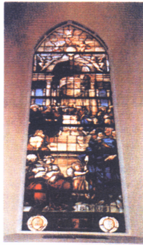
Fig. 1 Arrigo Fiammingo's window in the Cathedral of Perugia in its current state, with forced ventilation system in the space between artistic and protective glass
