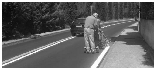
Figure 6: installation of paint stripes.
