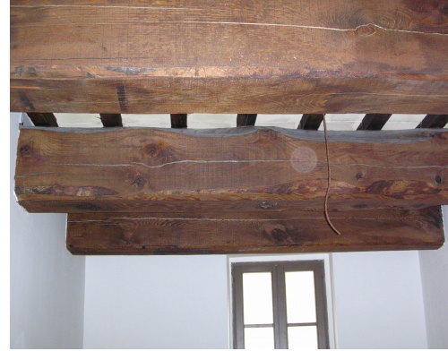
Figure 4: Wooden beam floor Particular of wooden beams
